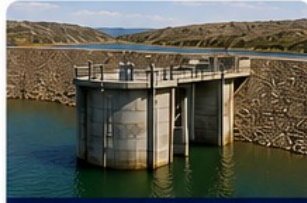
WATER INTAKE STRUCTURE
